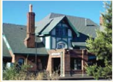
Flagstaff Visitor Center in the Historic Train Station
