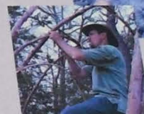
Strands of bark were used to tie the saplings together.
